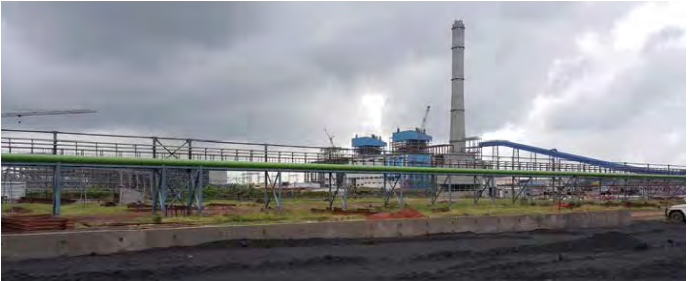
→ Haldia Project in progress
